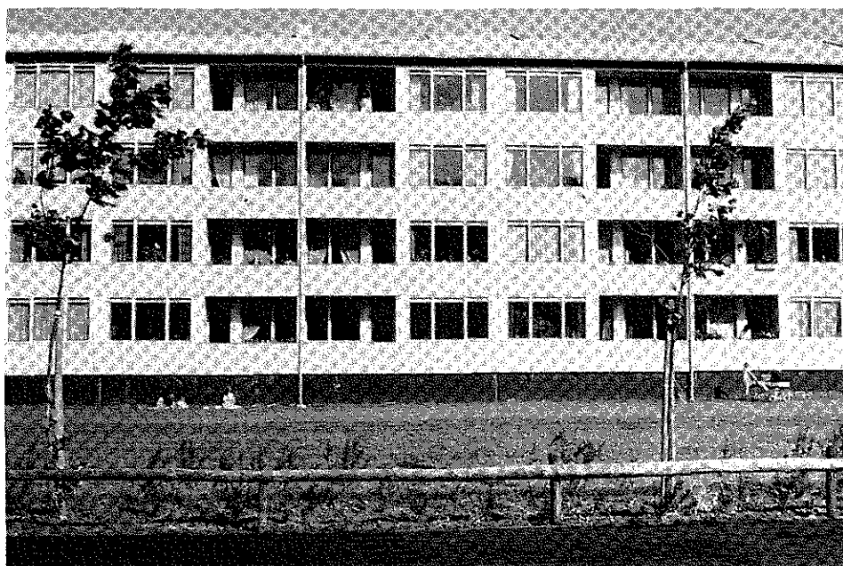
Figur 11.01. Altanfacade i Ballerup- planen. ★ Balcony facade in the Ballerup project.
