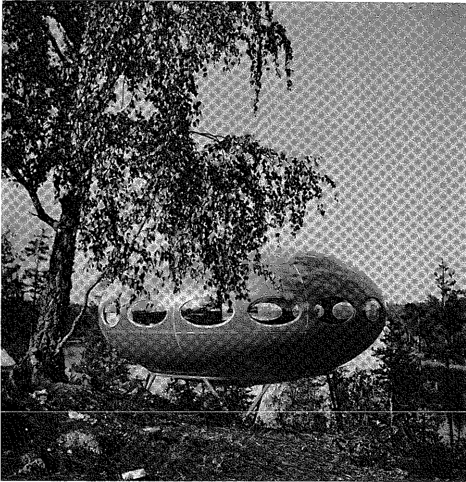
Figur 13.07. Det finske fritidshus „Futuro” af glasfiberarmeret polyester. ★ The Finnish weekend-house „Futuro” made of glassfibre reinforced polyester.
